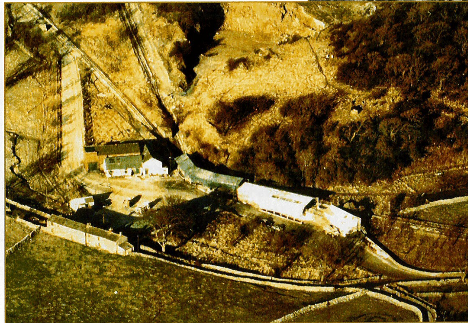
Fig. 18 Buildings at the junction of the inclines to the kilns (top left) and the tramway to the railhead in Threshfield. This is the modern entrance to Threshfield Quarry, seen here in the mid-1960s before the approach road from Threshfield was widened (bottom right).
