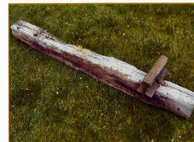
Fig. 20 A wooden sleeper and section of iron rail from the tramway.
