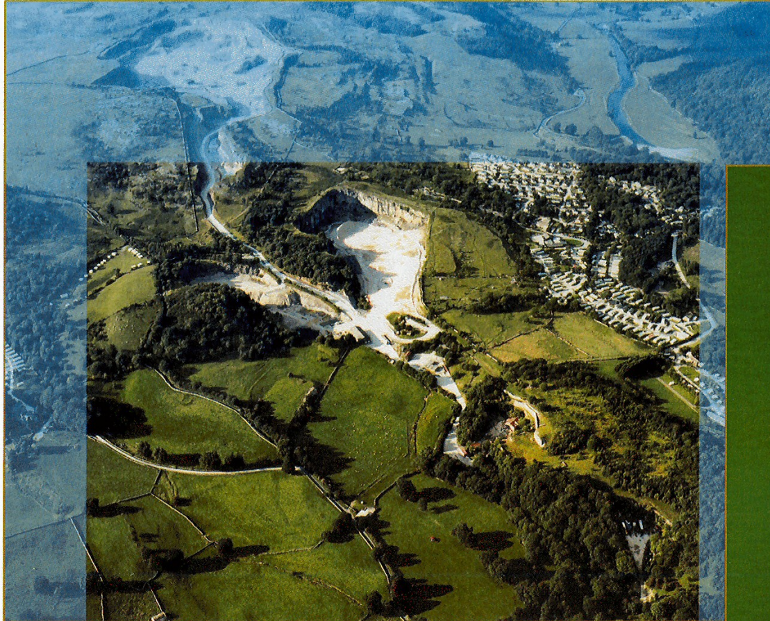
Fig. 9(a) Aerial photograph of Threshfield Quarry in 2004 © Tarmac Ltd.
