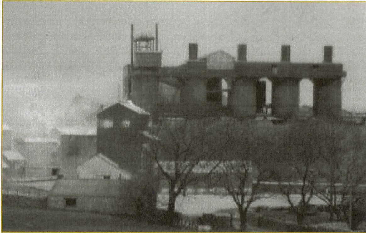
Fig. 6 The Spencer kilns at Threshfield Quarry in 1963.
