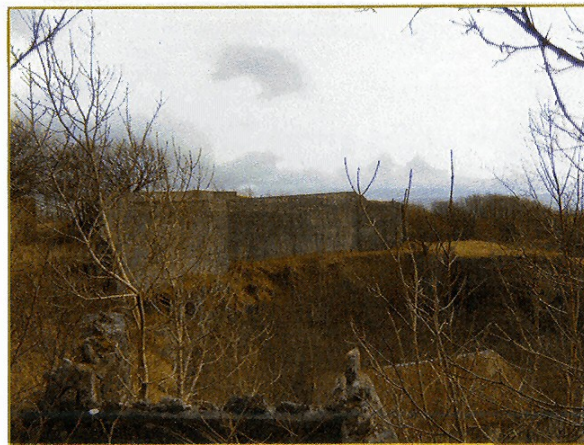
Fig. 21 The kiln superstructure in 1963 (l) and the brick buttressing that remains in 2008 (r). The 2008 view is taken across the 'Brown Hole', one of the original quarries.
